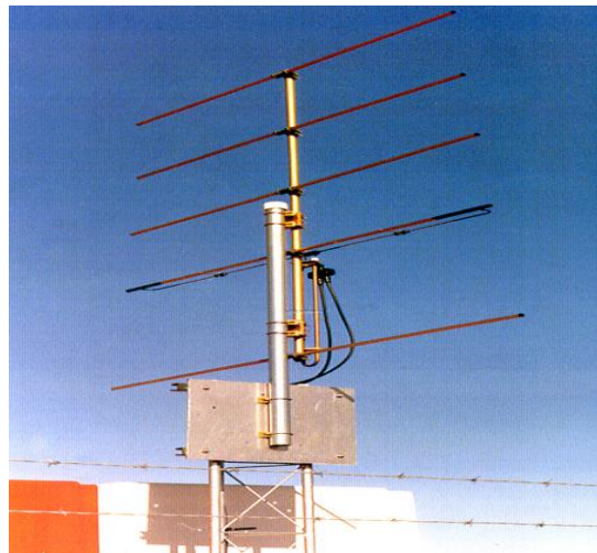
Figuur 23: Middle Marker antenne
